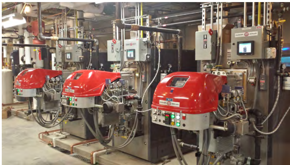
Pictured above are the three (3) TC600GO gas/oil Condensing Hot Water Heating Boilers that were installed at St. Lukes Fruitland Hospital in Fruitland, ID.
