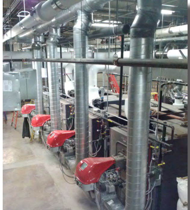
Pictured above are four (4) TC1450GO gas/oil Condensing Hot Water Boilers installed at Wayzata Central Middle School.
