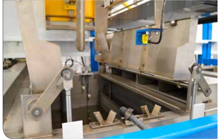
Every tank has sensors that autofill if needed, plus monitor the recirculation and filtration systems.
