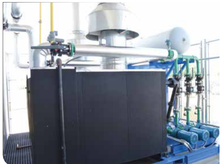
Ruger went with a different heating system than the gas-fired tanks it had; CJI brought in Parker Boiler for the project.
